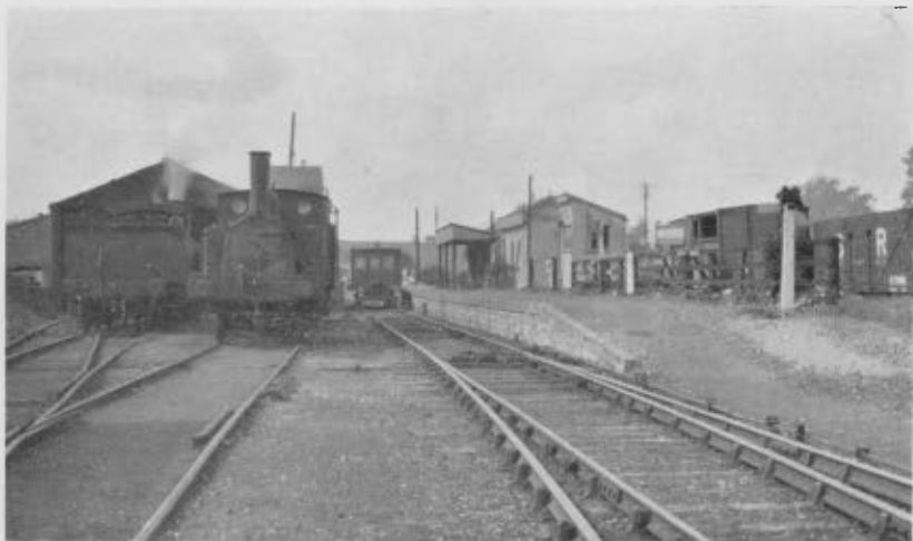
L.G.R.P. 7045. No. 1 "Tenterden," No. 9 "Juno" and Ford Railcar at Rolvenden Station.
